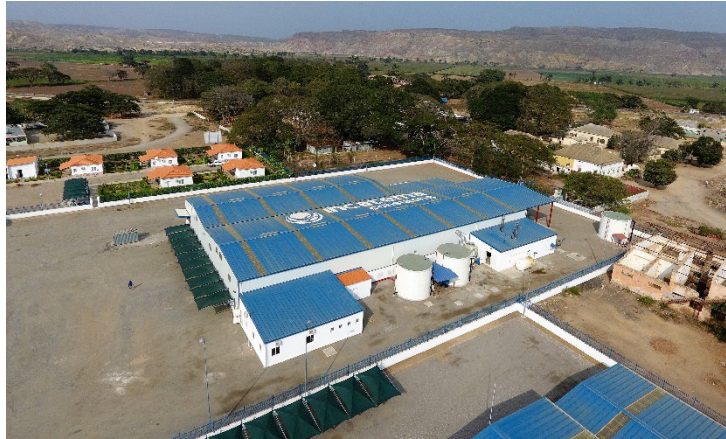
Tomato processing plant in Benguela, Angola
