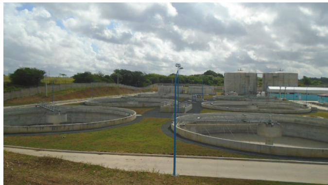
Ozama River wastewater treatment plant in Santo Domingo, Dominican Republic.
